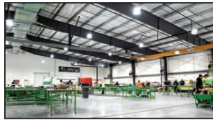
Game Composites is building the GameBird in a new, Modern facility at a quintessential GA airport in Bentonville, Ark. (Courtesy Game Composites)
